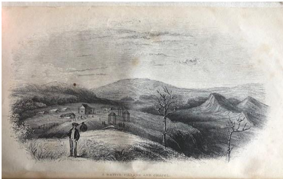
A native village and chapel. Marshall, 1834, frontis. In Yate it is labelled North-east view of the Waimate.
