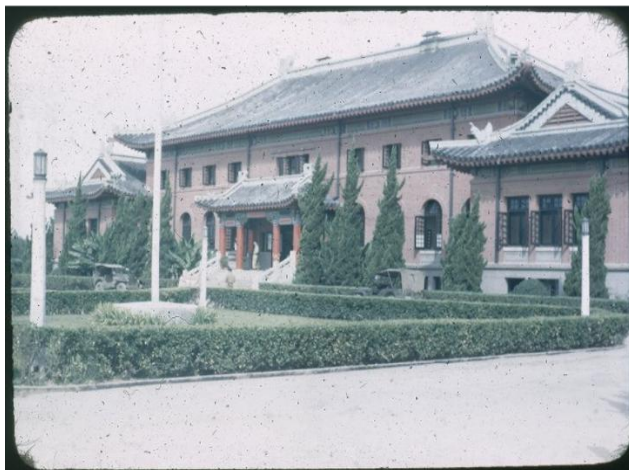
The entrance and part of the grounds of the Moral Endeavor Association Building (Li zhi she) in Nanking, 1945. Martin Hiller 1945. Hiller Collection, University of Missouri.
